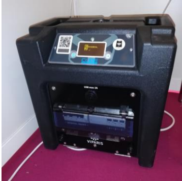
POWER SUPPLY (power ≤ 20kW)
